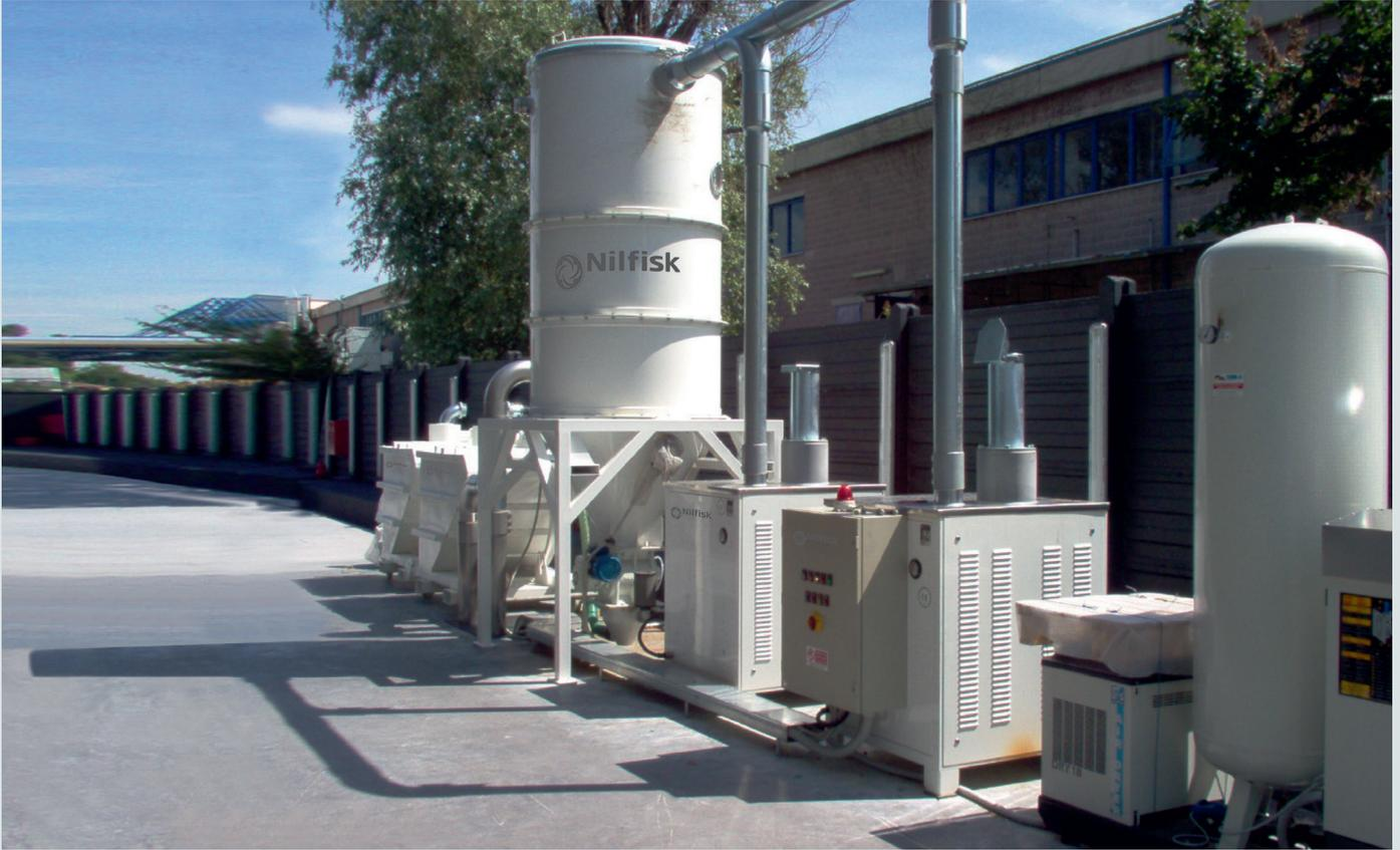
**Pneumatic conveyors** are an effective method to move dust and granules. They automate production, moving dust or granules from containers to machine tools. Employed to feed mixers, reactors, vibrating screens, granulators, capsule machines, compressors and blistering machine, pneumatic conveyors speed up the production process maintaining an healthy and safe environment.
